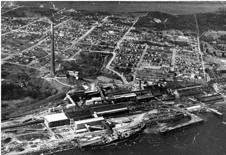
Figure 3. ASARCO Tacoma smelter. Left : Custodis stack, 573 ft. high, the tallest stack in the world at the time of its construction. Photo from the collection of Karen Pickett, Ruston Home blog.
